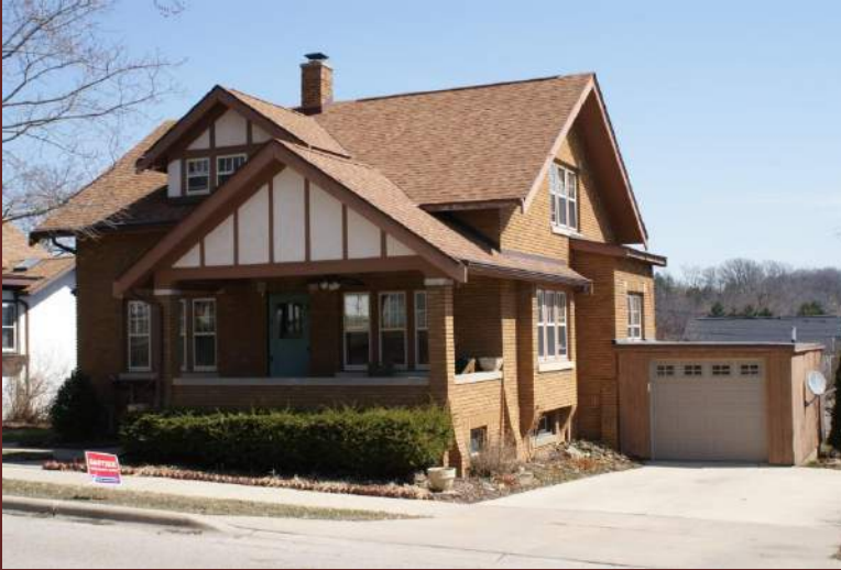
John Duerst House, 612 2 nd Street, 1927, Builder: Oswald Altman
