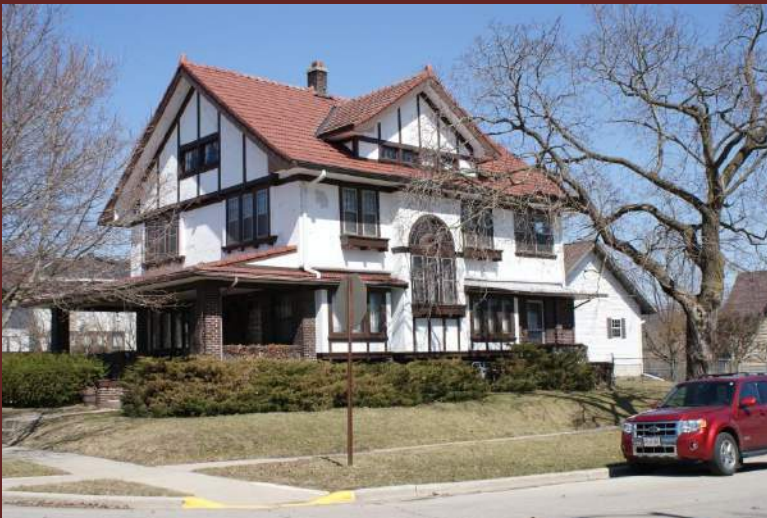
Dr. E. D. McQuillan House, 122 2 nd Street, 1913, Builder: Oswald Altman
