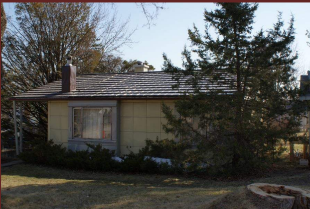
Lustron House (Walter Taplick), 419 8th Avenue, 1949
