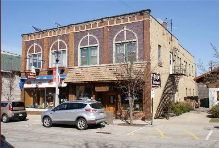
Albert Wolf Block, 534-538 1 st Street, 1916, Builder: Oswald Altman
